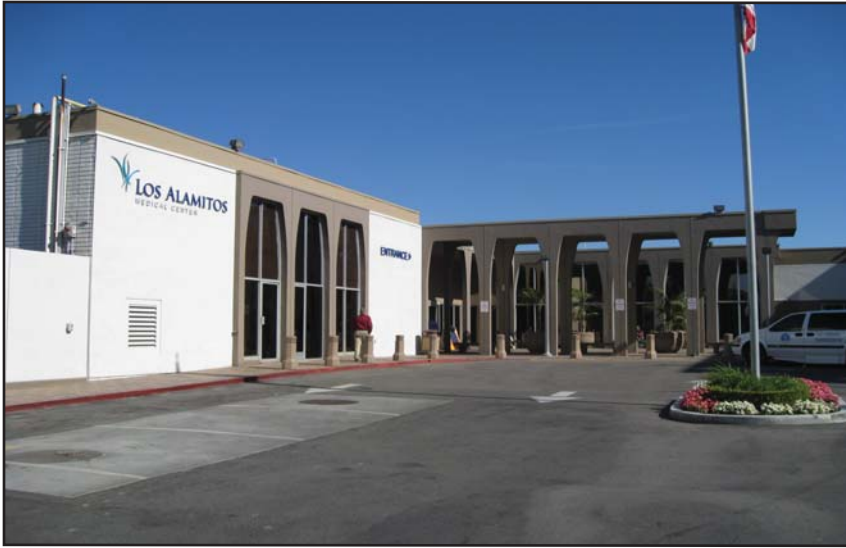
View of existing Main Hospital building (3751 Katella Avenue).
