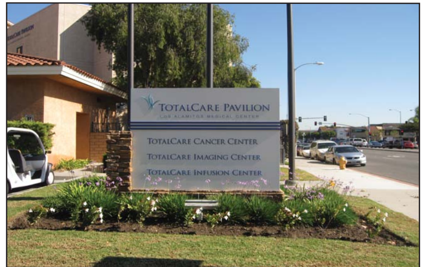
View of existing Total Care Pavilion (3951 Katella Avenue).
