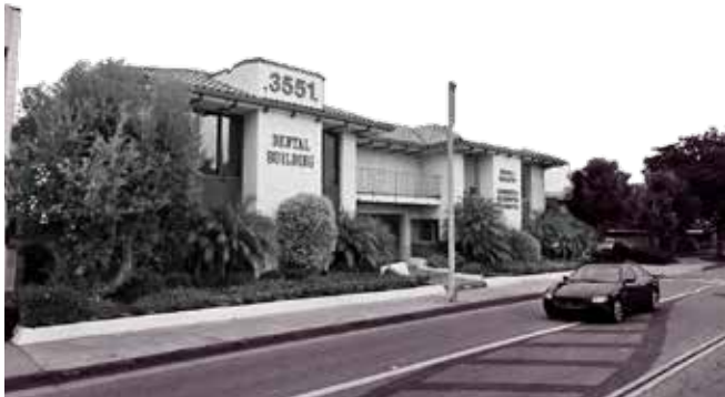
Two and three story medical offices are a prominent and stable land use within the Plan Area.
