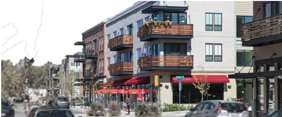
Ground floor retail and restaurants with residential units above.
